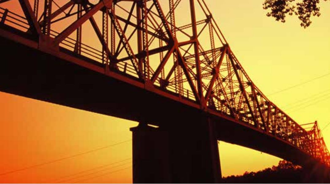
Photo courtesy of the Arkansas State Highway and Transportation Department
