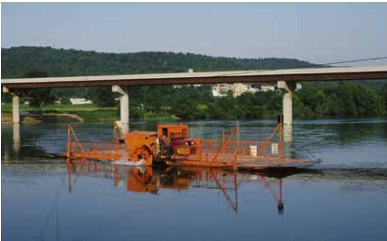
Photo courtesy of the Arkansas state Highway and Transportation Department
